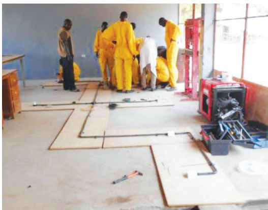
Students conducting a full conduit wiring
